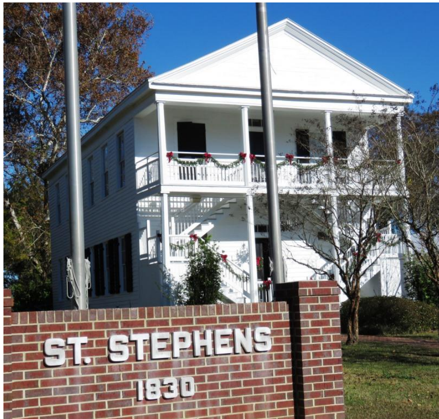
The ex-Courthouse/ex-Masonic Lodge and current OSS Museum at (new) St. Stephens
